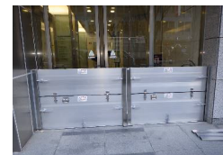
Installation of flood barriers (NBF Higashi-Ginza Square)
