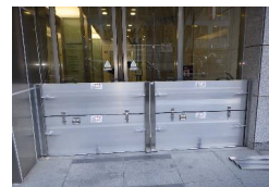
Installation of flood barriers (NBF Higashi-Ginza Square)
