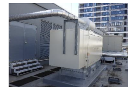
Inspection/update of emergency power generator (NBF Takanawa Building)
